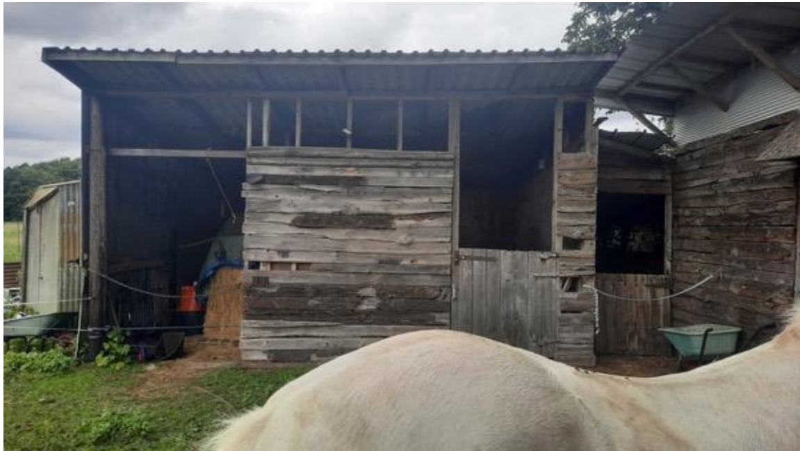
Photo 14. Wooden stable building in northwest corner – southern section
