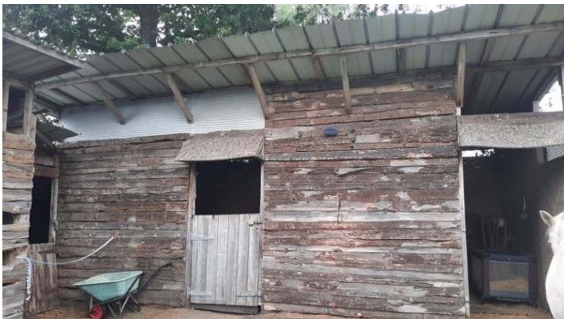
Photo 15. Wooden stable building in northwest corner – northern section
